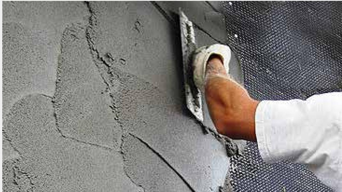
Sienna Wall Float is a mortar consisting of portland cement complying with ASTM C150, hydrated lime complying with ASTM C207, and sand complying with ASTM C144. Sienna Wall Float is designed to be used as a scratch and brown coat for most tile and stone installations. Flexibility, adhesion, and water resistance of the wall float are improved when Sienna Admix AX300 or AX400 are used in lieu of water. Sienna Wall Float is available in grey in both 50 lb and 75 lb bags.
